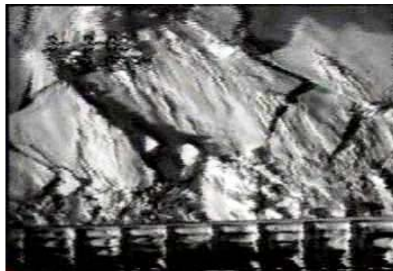
Figure 2 A view of a first year ridge interaction on the west side of the caisson, taken from the derrick top camera on March 3, 1986. The ice deflector is in the foreground.
