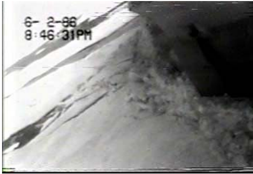
bending and splitting failures along the east face of the caisson
